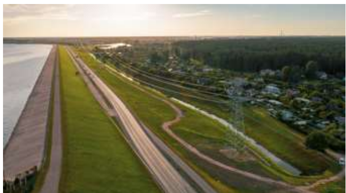
Fig. 9. 330 kV electricity transmission line Riga CHP-2 – Riga HPP
